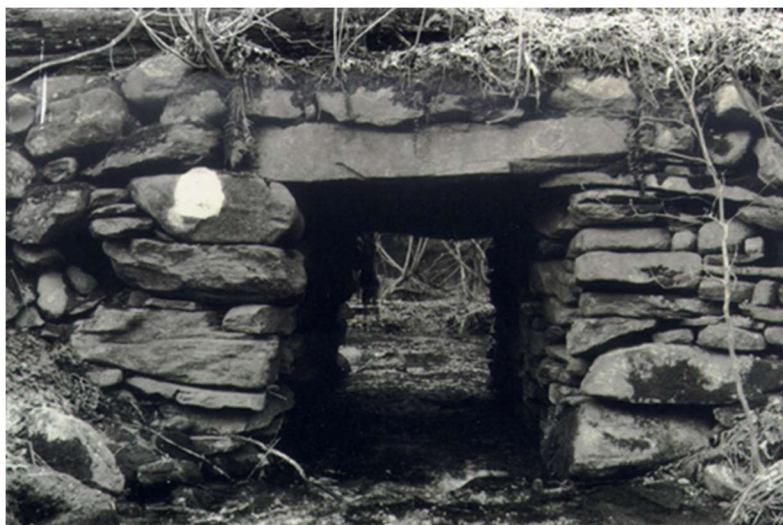
A traditional stone culvert. Still in use on Deer Ridge Road, off of Route 35. (G)
